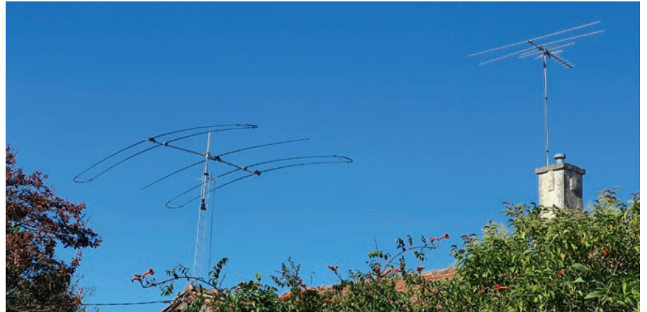
Fig.13 (below): David's Yagi antenna (on the left; the TV antenna on the right is also a Yagi).
